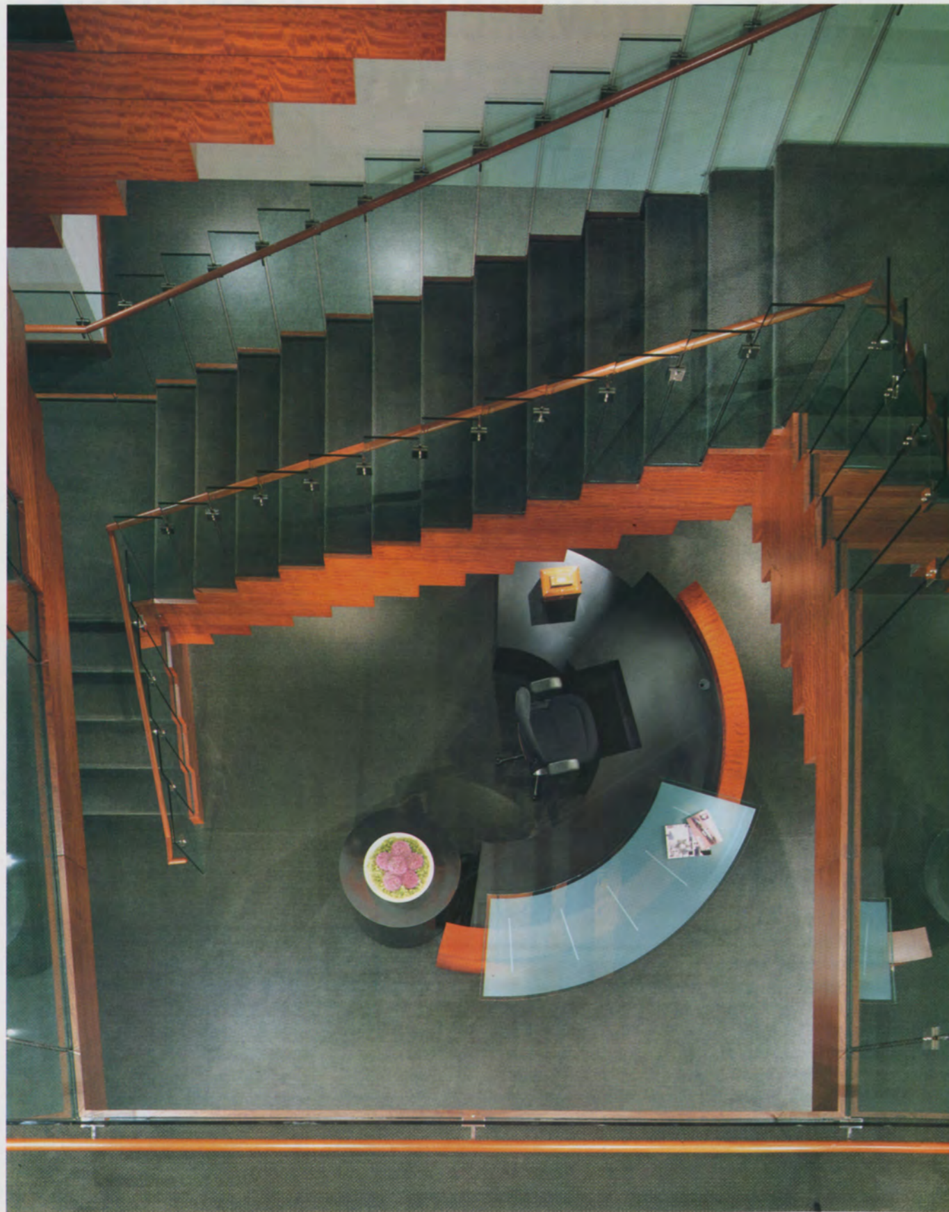
A view of the spectacular four-story stair system with the reception desk at the bottom. All exposed surfaces of the stairs were wrapped in veneer panels except for the treads and risers. All veneer is quartered figured Sapele.
