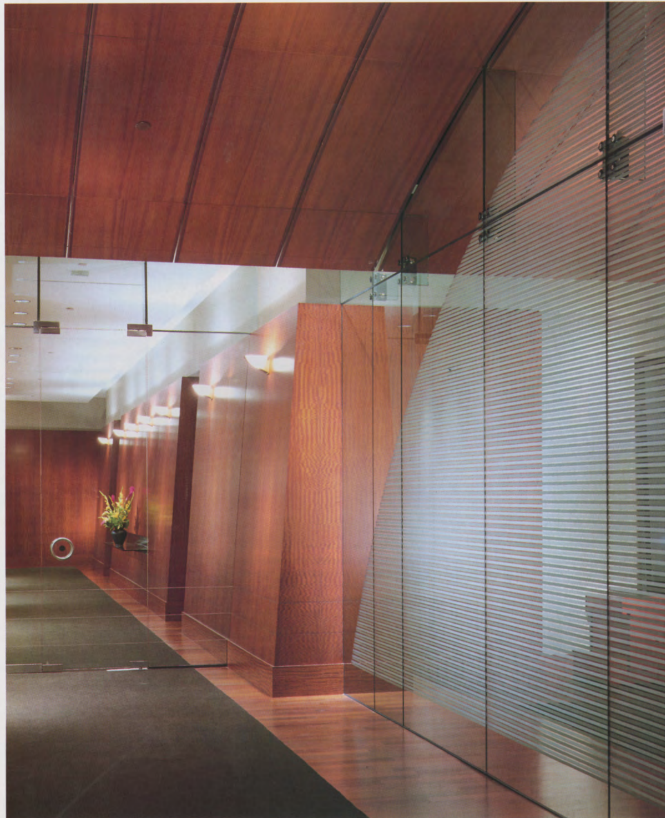
The elevator lobby canted wall and the vaulted ceiling created some challenges for the woodworker. Veneers are quartered figured Sapele on the walls and figured plain sliced Makore on the ceiling.
